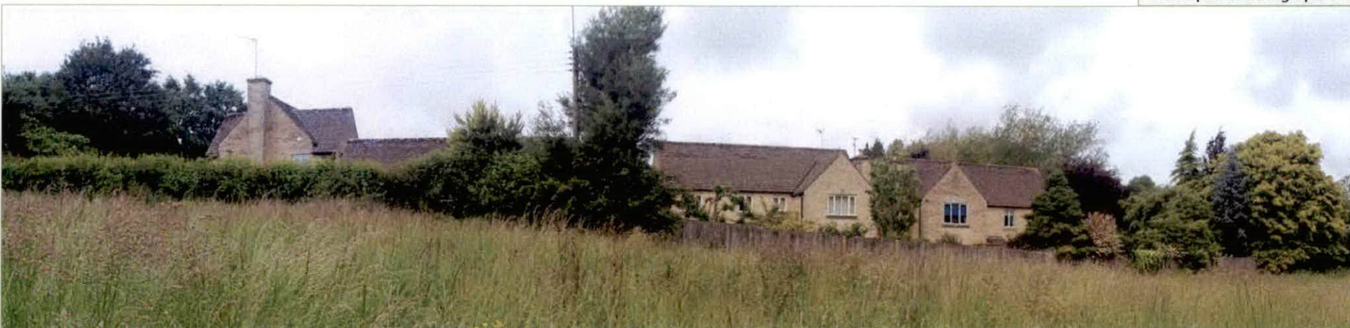
View looking west into site from eastern boundary
